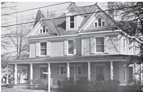
In 1905, Mena Ray and Lucius Glenn built this impressive 3,352 square foot home across the street from his parents' home. It still stands at 402 South Chester Street, Gastonia. Courtesy of Gaston County Historic Properties Commission.
