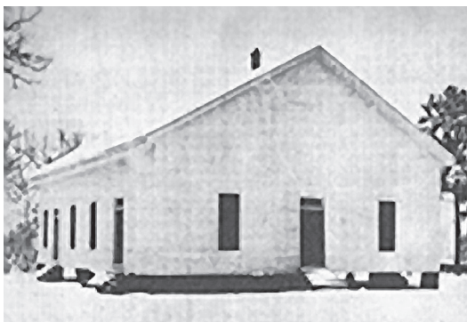
Olney Independent Presbyterian Church was the church home of several generations of Torrence and Wilson families. Used with the permission of Olney Presbyterian Church.
