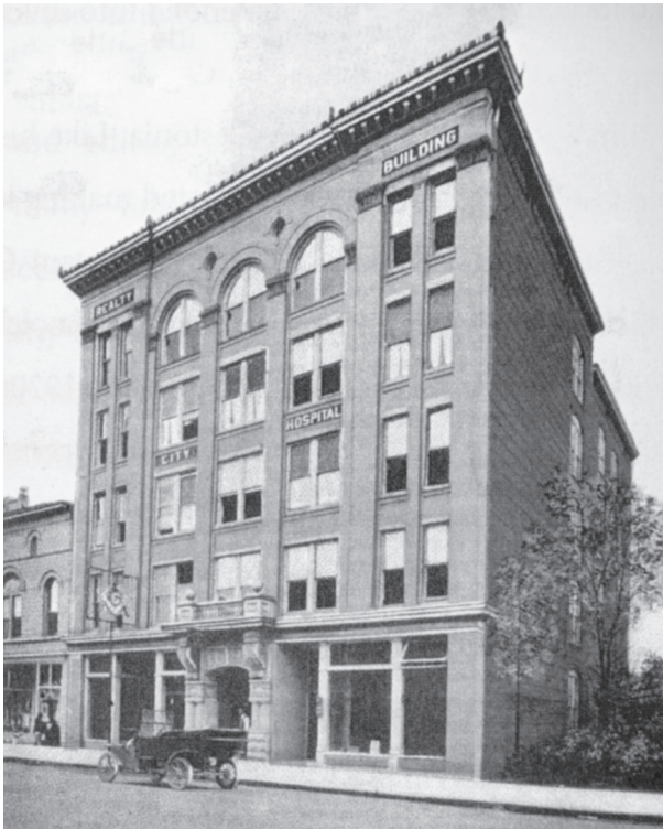
City Hospital’s second location was in the new Realty Building on Main Street. The hospital occupied the third, fourth, and part of the fifth floors. Courtesy of Robert Allison Ragan.
